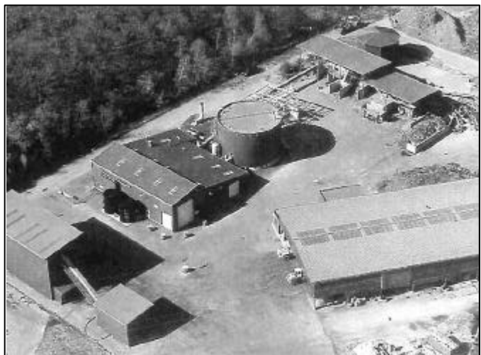
Figure 6: The VALORGA-plant of Bernex, Geneva: A cylindrical digester with a volume of 1000 m 3 treats easily digestible wastes on a composting plant.
